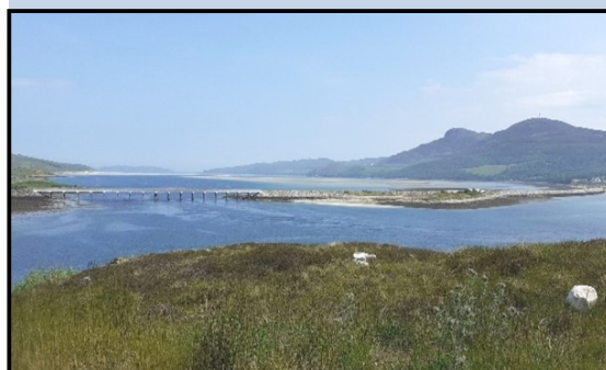
Kyle of Tongue Road Bridge
